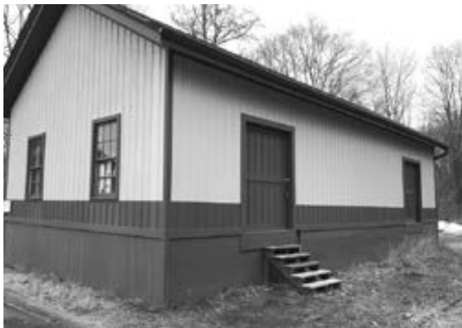
The freight house doors are at the same level as boxcar doors. The stairs shown here are of recent date. Originally there was a long, wide loading platform at door height, located between the freight house and the boxcars on the adjacent siding. It was big enough to hold a lot of freight shipments. (Photo by Paul Penfield Jr.)
