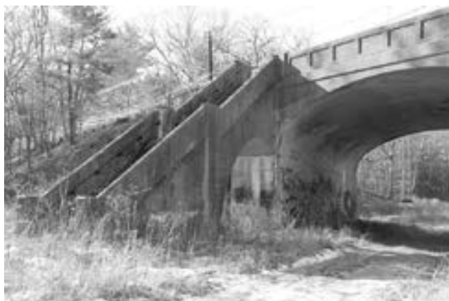
The Church Street bridge has a very unusual shape. First, it has two arches. The larger one is wide enough for two railroad tracks and the smaller one for vehicle access to the freight spur track. Secondly, extending out from the east side it has a stairway resembling a buttress, connecting to the Church Street sidewalk. (Photo by Valerie Mertz).
