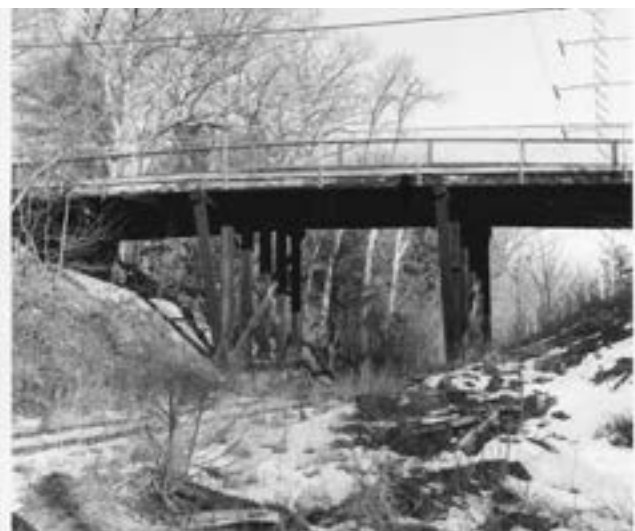
Looking east at the Conant Road bridge in January 1988, five months prior to its demolition. The high elevation in the middle blocked motorists' views of oncoming traffic. Wooden bridges are more suitable for roads without heavy truck traffic. The truck weight limit on this bridge was about four tons per axle. (Photo by R. Richard Conard)
